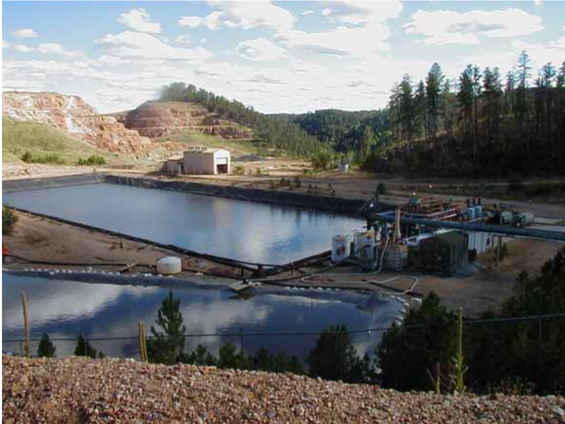
Figure 8. On-site Treatment of Acid Mine Drainage
