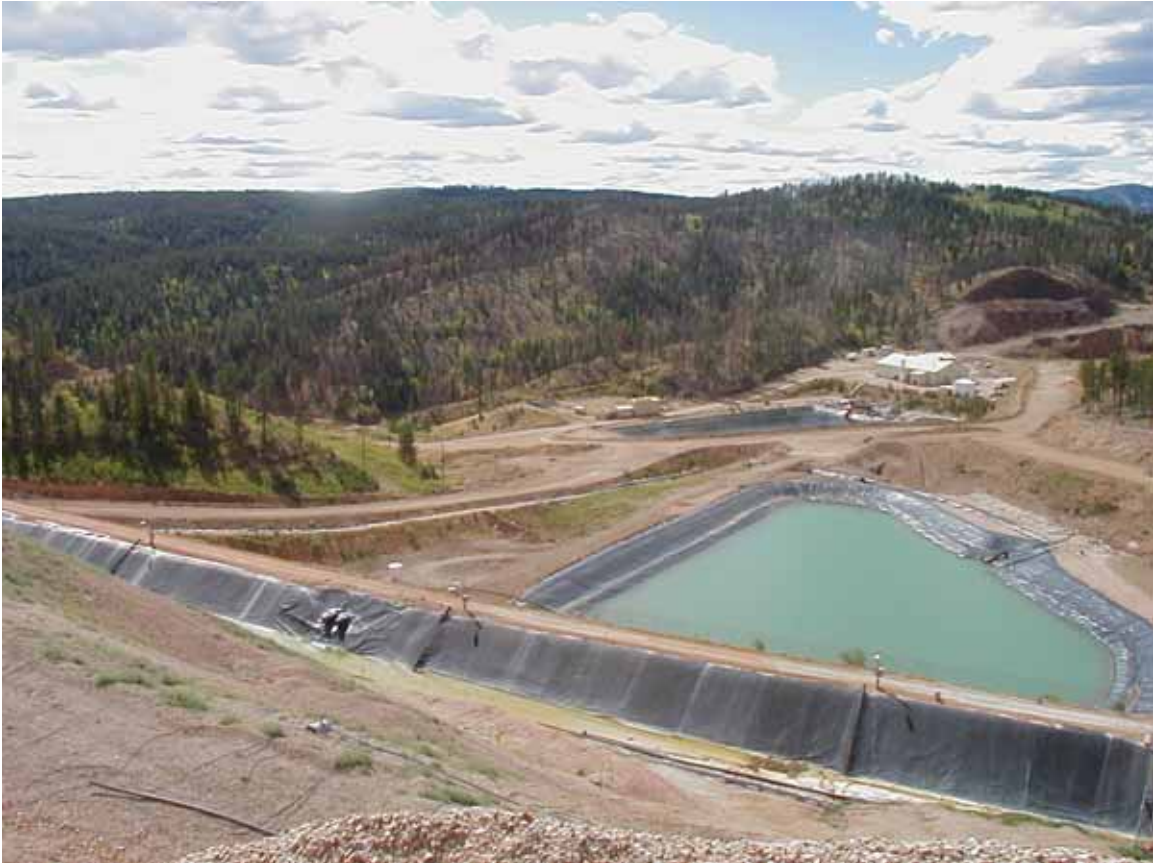
Figure 5. On-site treatment of acid mine drainage.
