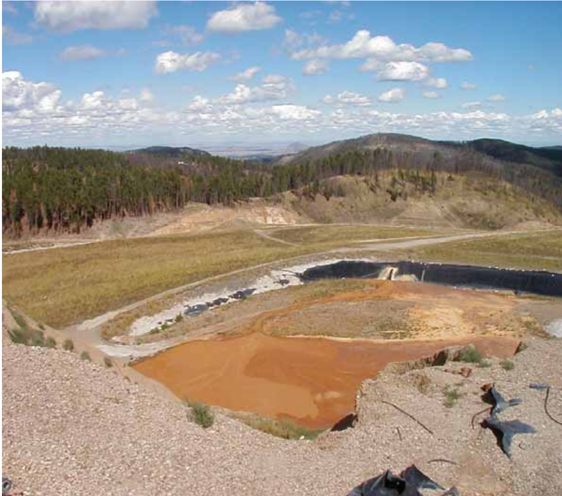
Figure 4. Sediment retention pond for heap leach pad and portion of Ruby Gulch Waste Rock Cap.
